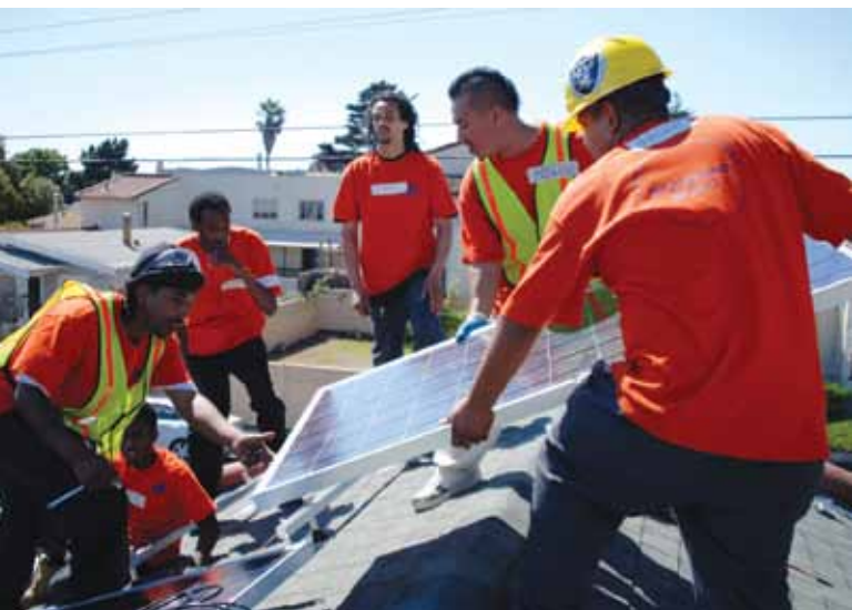
Workers in the "Solar Richmond" training program install solar panels
