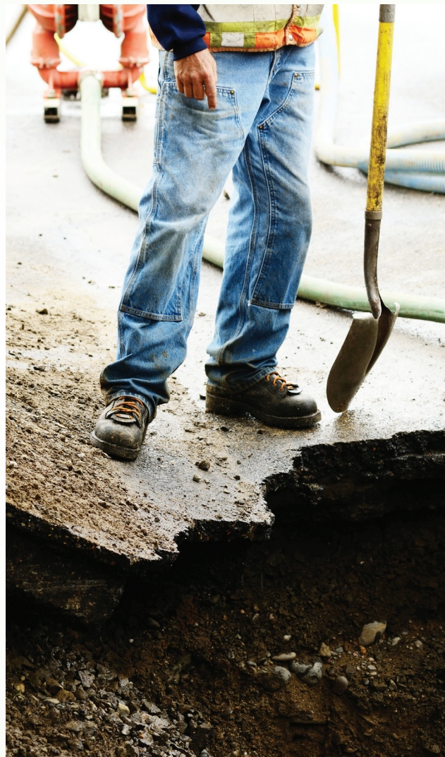
Photo: a worker fixing a water main break. The EPA estimates that there are 240,000 water main breaks per year in the United States.
